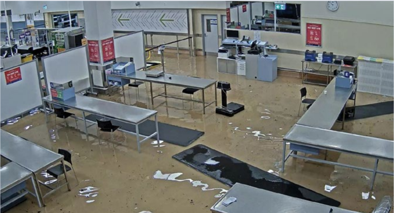
Customs Auckland International Airport search area flooding on 27 January 2023.
